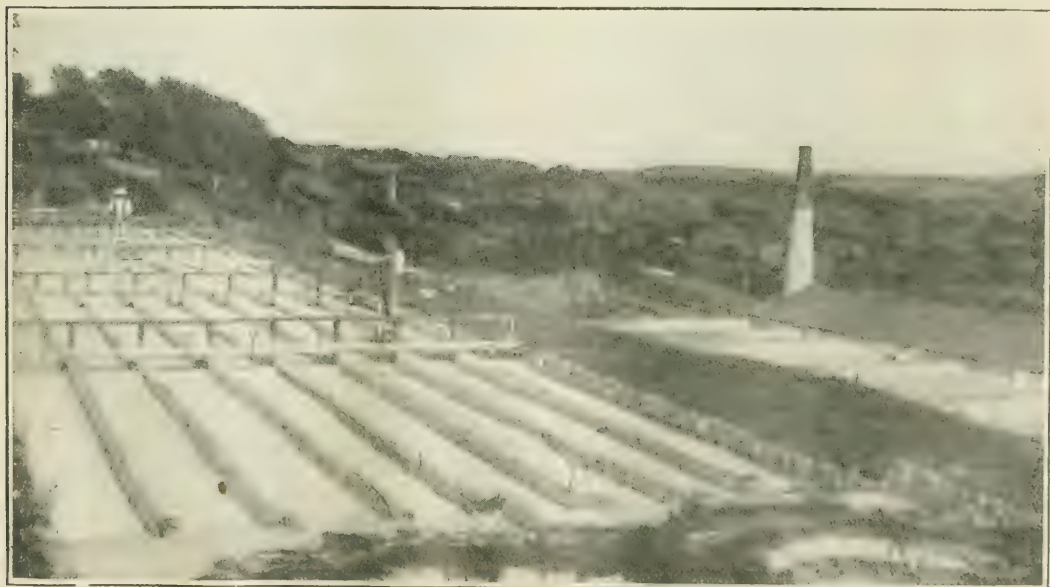
FIG. 6. OLD-FASHIONED "MICAS" BUILT OF STONE. (Photo, English China Clays, Ltd., St. Austell).
